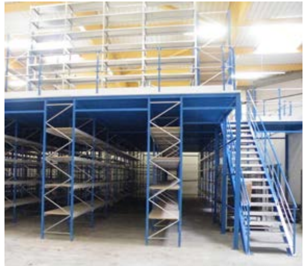
Mezzanine over Epsivol shelving.
